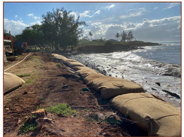
After the sandbag structure being repositioned and new bags added.
